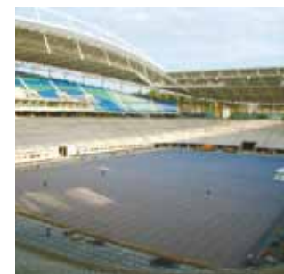
Undersoil pitch heating
